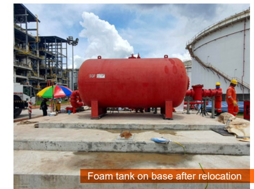
Foam Tank Relocation Work - Lifting Activities
