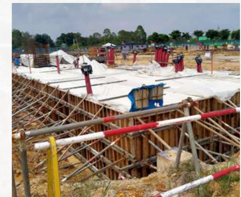
Gas Turbine Generator #2 foundation (curing)
