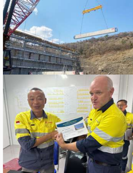
Congratulations to Liang Xiao who successfully set in motion the idea of using pre-cast to significantly reduce the weeks required to cast roof beams on the Gas Insulated Substation.
