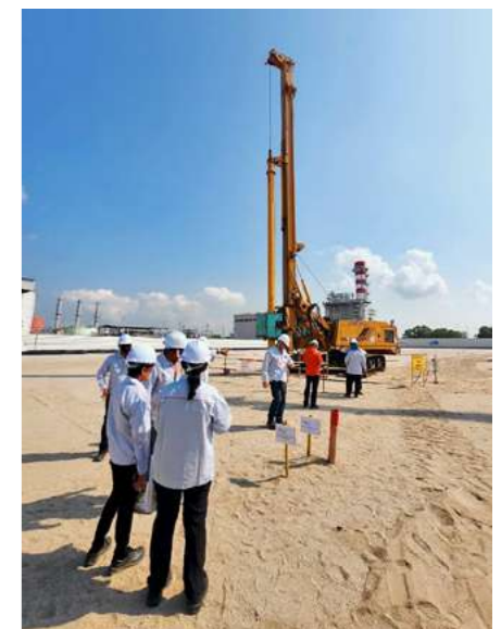
Bore pile rig is assembled and testing in progress.
