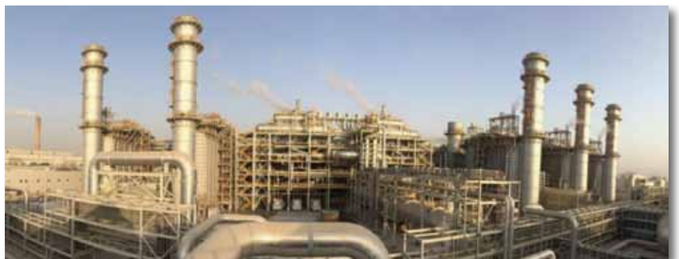
▲ Front view of HRSG (5 units) with STG #16 & 17 interconnected power block pipe rack
