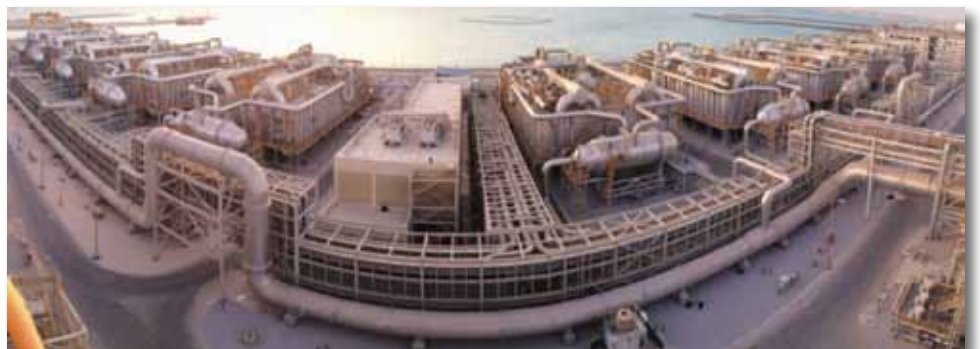
▲ Front view of HRSG (5 units) with STG #16 & 17 interconnected power block pipe rack
