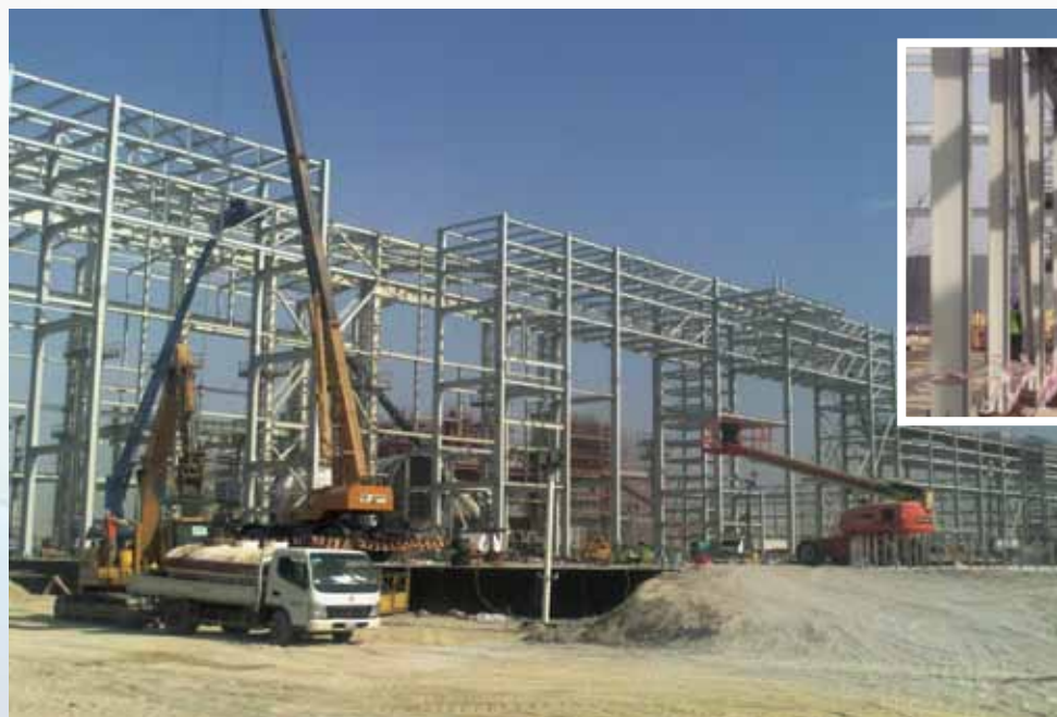
Main Rack #2 Structures Installation
