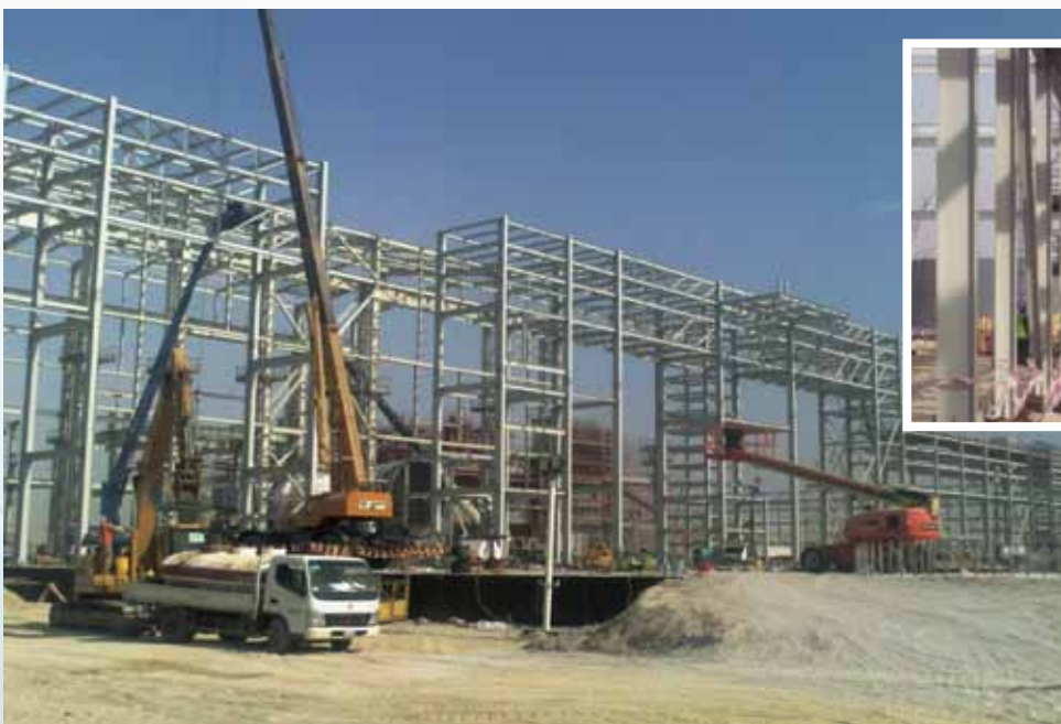
Main Rack #2 Structures Installation
