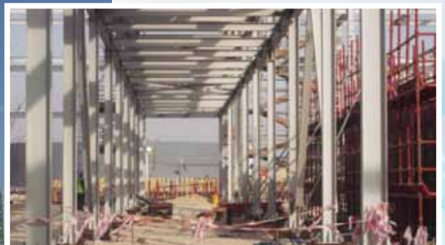
WTR - II Pipe Rack Structures Installation
