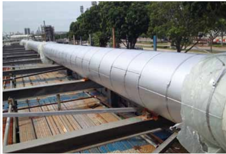
HP Steam Line Installation
