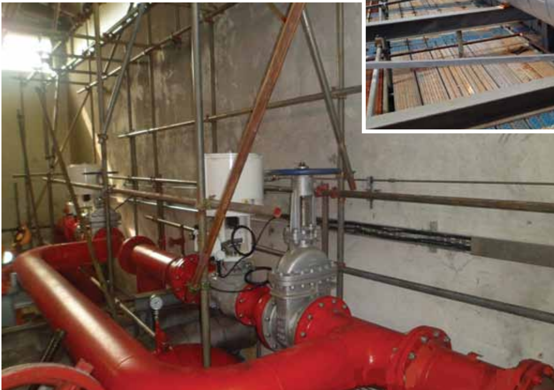
Sereya Fire Water Pump House Piping & PCV Installation
