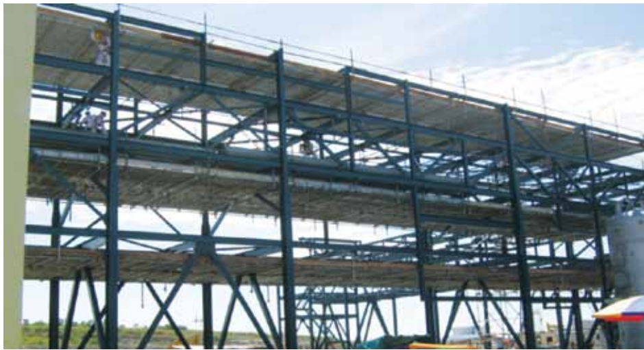
Pipe Rack Piping Installation Work - Pipe "Launching" @ Erected Pipe Rack
