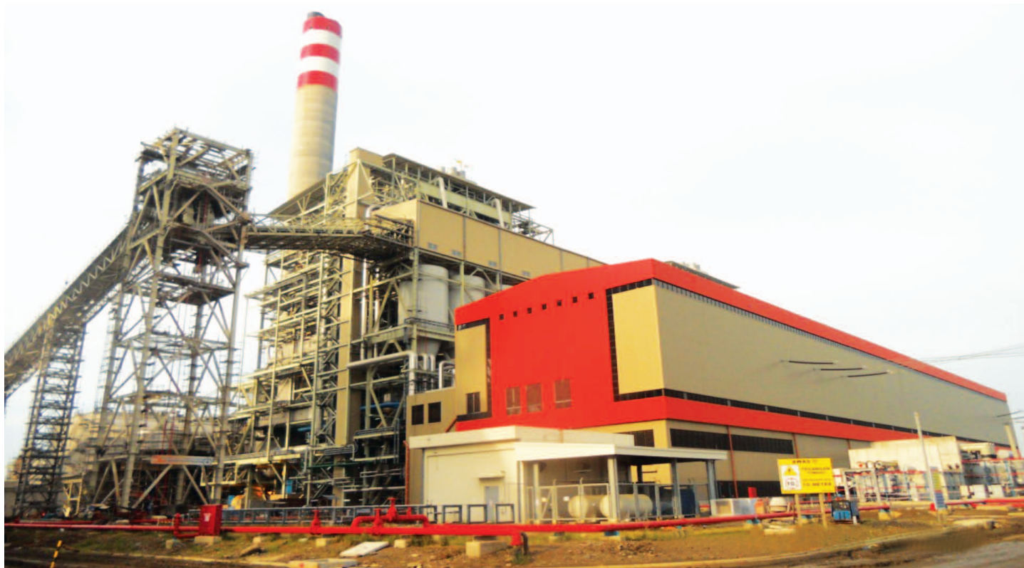
Tanjung Jati “B” expansion project unit #3 – boiler and turbine building
