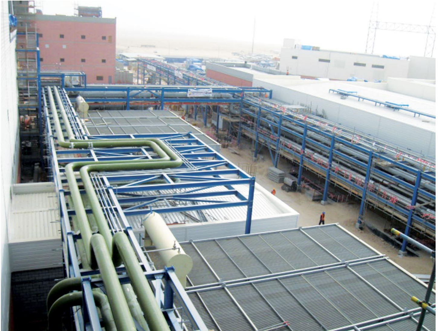
Pipe Rack Steel Structure and Piping Installation at the Sabiya CCGT plant
