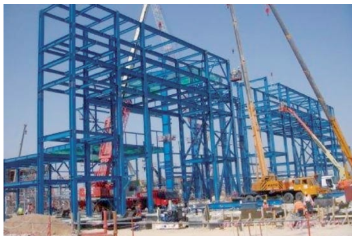
Sabiya CCGT Project – Erection of Pipe Rack Steel Structures in progress
