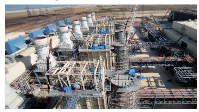
Aerial view of HRSG's connecting to the turbine house through pipe rack.
