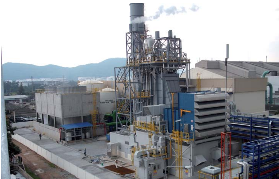
Overall view of Sime Laem Chabang Project in Thailand.
