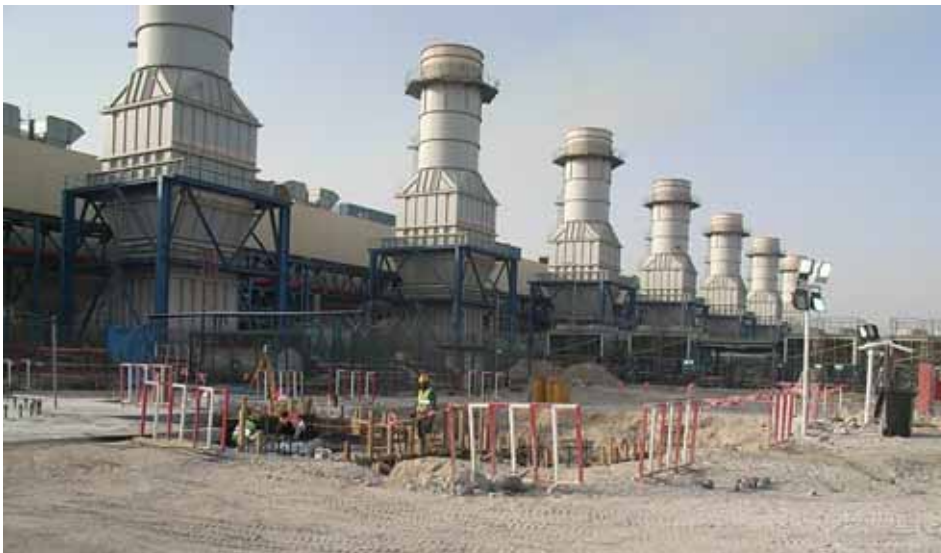
Overall view of the construction area for eight HRSGs.
