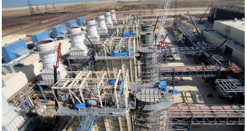
Aerial view of HRSG's connecting to the turbine house through pipe rack.
