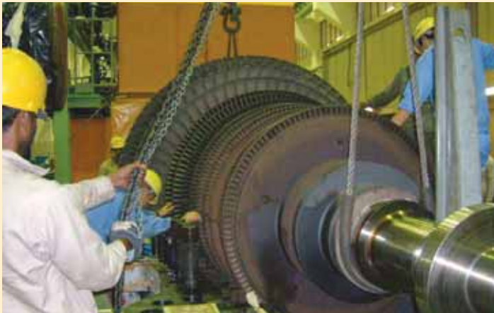
Turbine overhaul work in progress.
