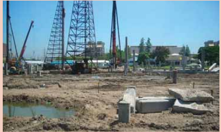
The plant is a 730-MW multi-shaft combined cycle generating unit.
